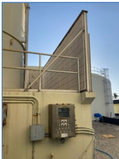
Replace Control Panel
